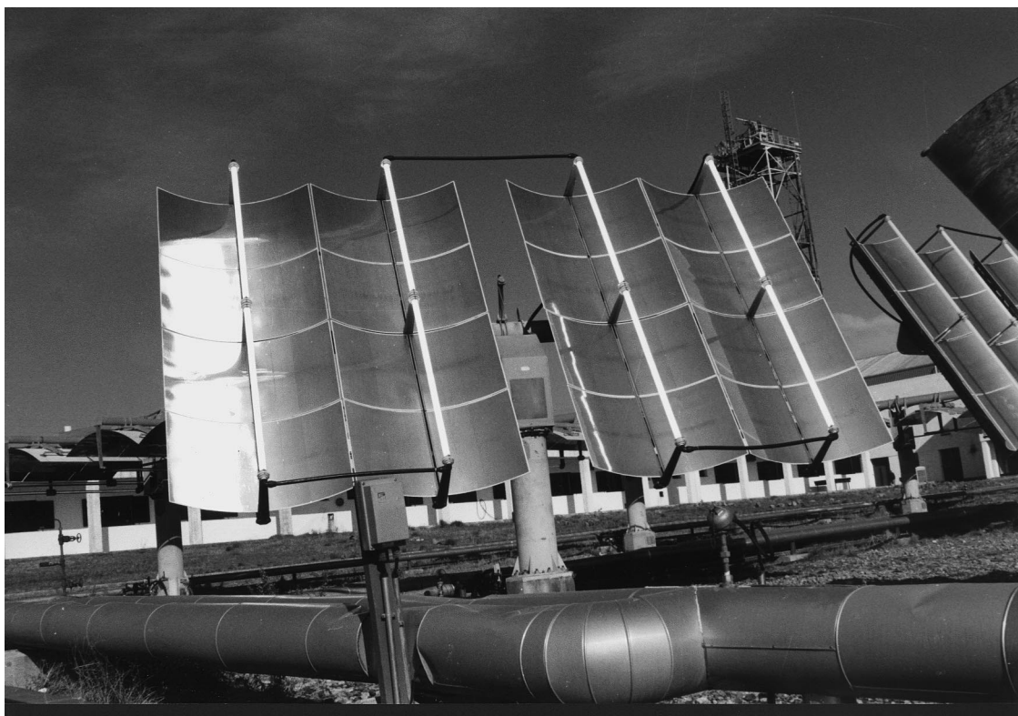
Fig. 6. View of a parabolic trough reactor, type “Helioman”, installed at the PSA (Photo: Goslich).
